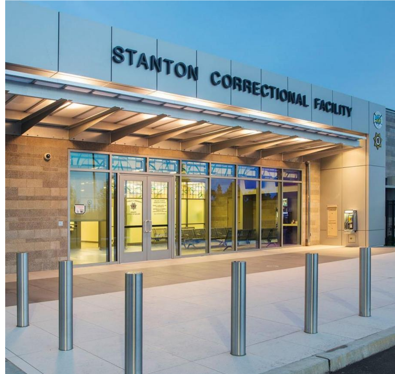
Sloan Programmed Water Technologies (PWT) Case Study: Stanton Correctional Facility, Claybank Adult Detention Center , Fairfield, California
